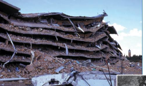
← Figure 36a: A strong, mining-induced earthquake in 1976 caused extensive damage (for example, the collapse of this six-storey high block of flats, known as the 'Tempest Hof' flats) in the town of Welkom, southwest Witwatersrand basin.
